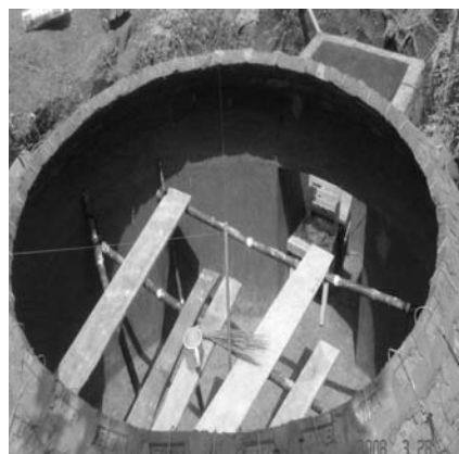
Biogas plant under construction
